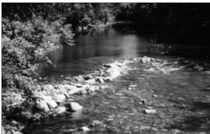
Rock vanes were built in the stream to reduce erosion.
